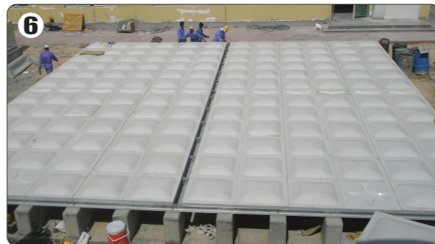
6 Assemble bottom panel
