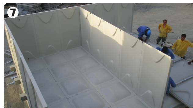
7 Erect wall and partition panel
