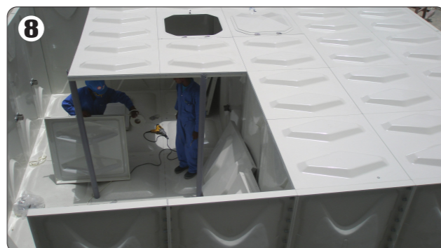
8 Assemble roof panel and manhole
