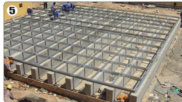
5 Concrete foundation for the erection of water tank
