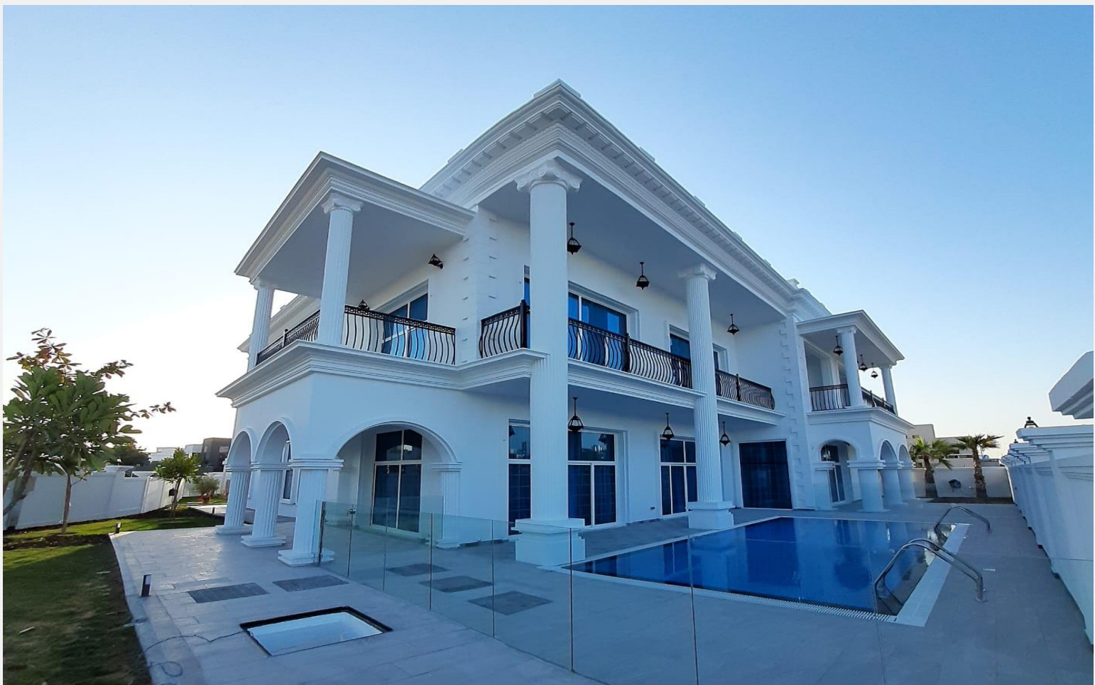
Project: PROPOSED G + 1 + R + SB Villa, Al Qouz 2, Dubai. Owner: Ahmad Bin Salmin Al Bebdawi Job: MEP Works
